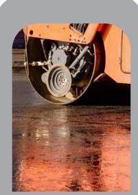
Boral's high-binder crumbed rubber asphalt surfacing integrates endof-life OTR tyres, sourced from quarry haul dump trucks and front-end loaders operating at Boral facilities.
