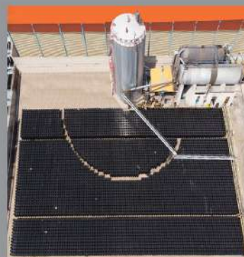
SEPAHAN BITUMEN JEY Isfahan - IRAN
